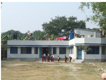
Bethel House with new coat of paint
